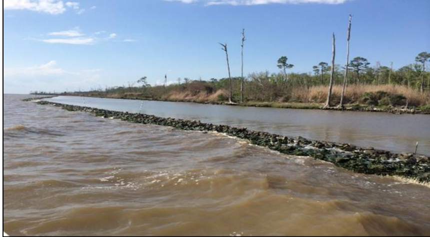
Figure 2 Living shoreline breakwater during MHW tide at Swift Tract in Bon Secour Bay, Alabama, showing wave reducing effects.
